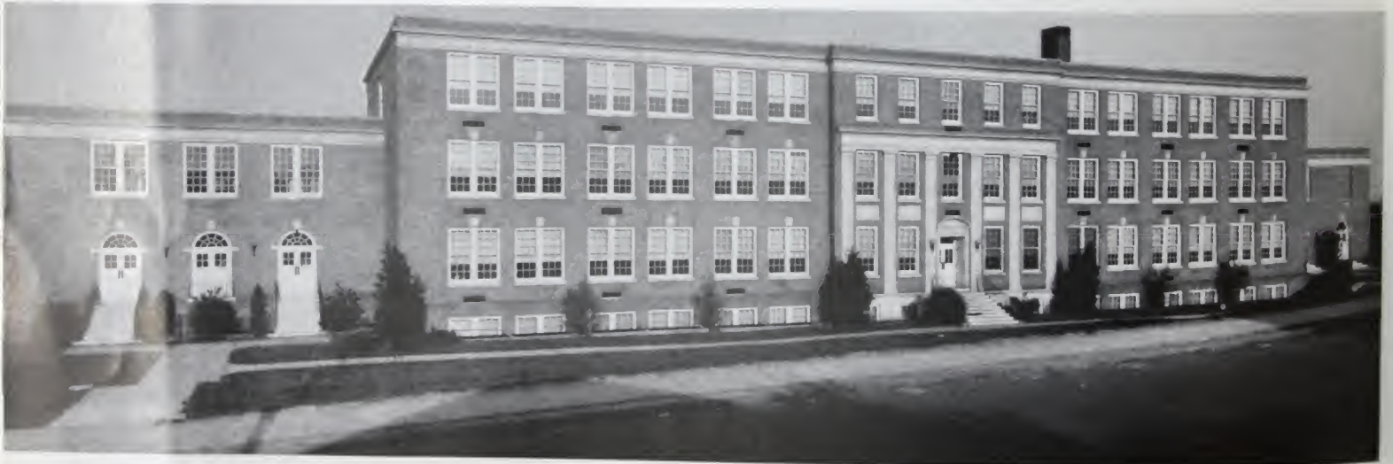
High School, Winston-Salem, North Carolina Harold Macklin, Architect F. L. Blum & Co., Contractors Standard Supply Co., Dealer Medusa Waterproofed Gray Portland Cement used.
